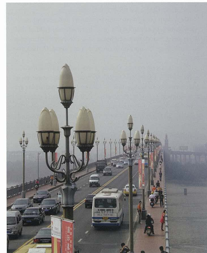
FIGURE 8. For readers with an interest in history: this looks like the classical photographs of 1970’s China except that the cars are modern. This is looking onto the top deck of the Nanjing Bridge, now supplemented by two others across the Yangtze River. The bridge was completed using Chinese technology after the Soviet Union walked away from the project as a result of a cooling of relations. The road lighting luminaires, in the form of closed lotus blossoms, were apparently designed by Zhou Enlai, China’s amazing Foreign Minister and stabilising element during the Cultural Revolution. In deference to him, they can be still seen in most major public spaces in China. They still adorn Tiananmen Square in Beijing.
